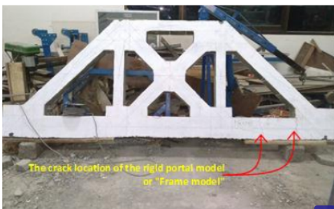
2 Fig. 8. The crack pattern of the rigid portal model or "Frame model"
