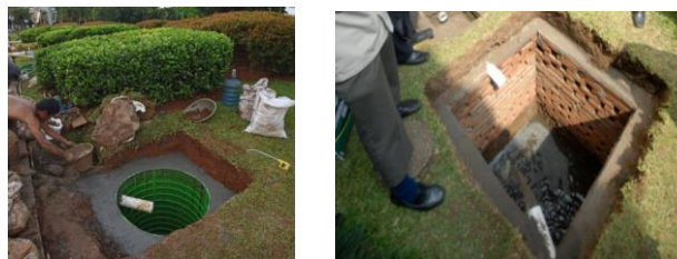
Figure 2. Prototype of infiltration wells in the field
