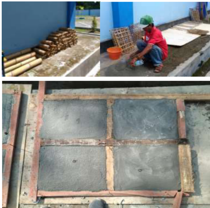
Figure 3. The process of drying reinforcement and preparation for casting
