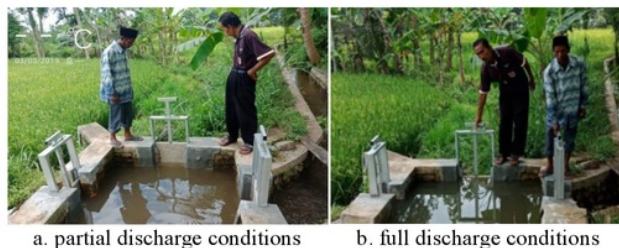
Fig 8. Test the sluice field of concrete panels
