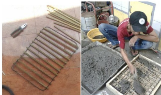
Fig 3. The process of making water gates from panels with reinforcement from bamboo
