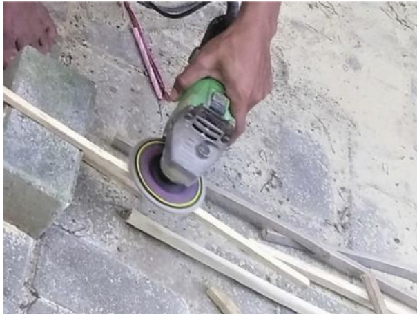
Fig. 7. Fireplace; treating the surface of bamboo reinforcement with a grinding machine.
