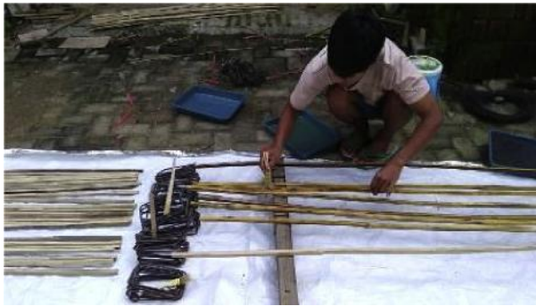
Fig. 9. The initial surfacing of Sikadur®-752 adhesive.
