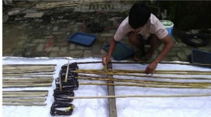
Fig. 9. The initial surfacing of Sikadur®-752 adhesive.
