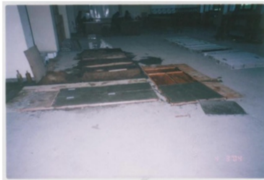
Fig. 4. Manufacture of panel test specimens
