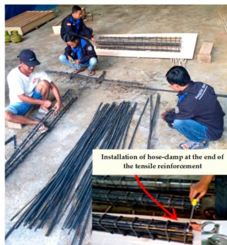
Figure 8. Stringing the bamboo reinforcement.
