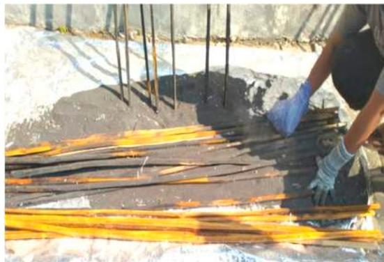
**Figure 7.** Sand sprinkling on bamboo reinforcement.
