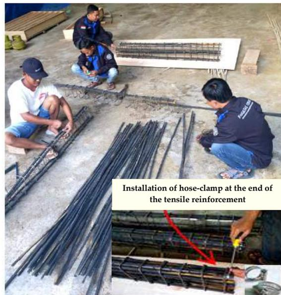
**Figure 8.** Stringing bamboo reinforcement
