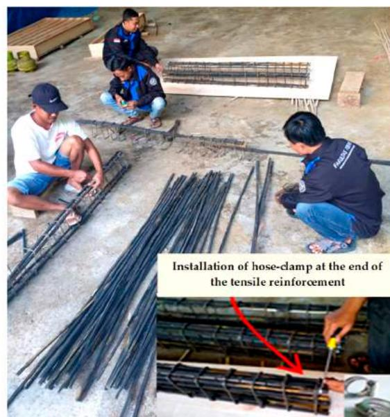
**Figure 8.** Stringing the bamboo reinforcement.
