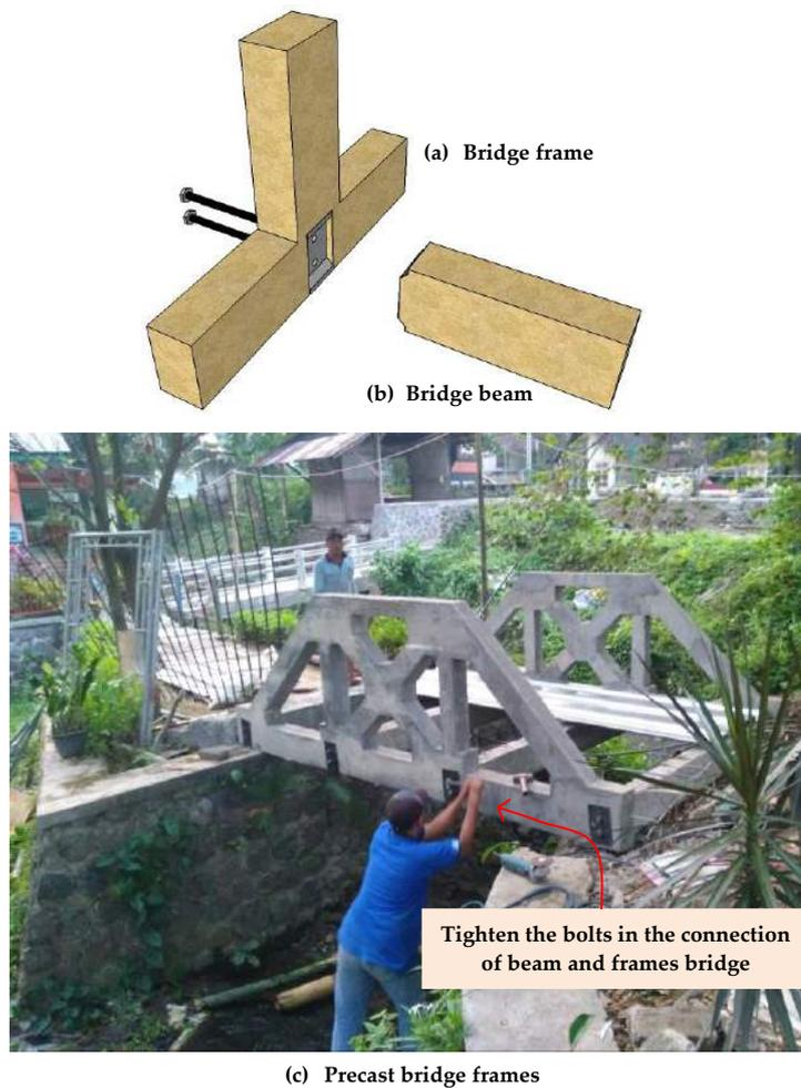
Figure 11. Models and applications of the precast connections.
