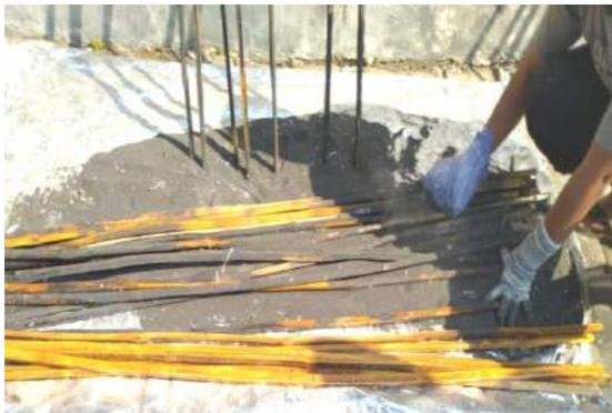
**Figure 7.** Sand sprinkling on bamboo reinforcement
