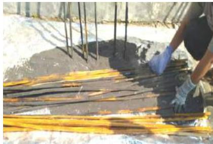
Figure 7. Sand sprinkling on bamboo reinforcement.
