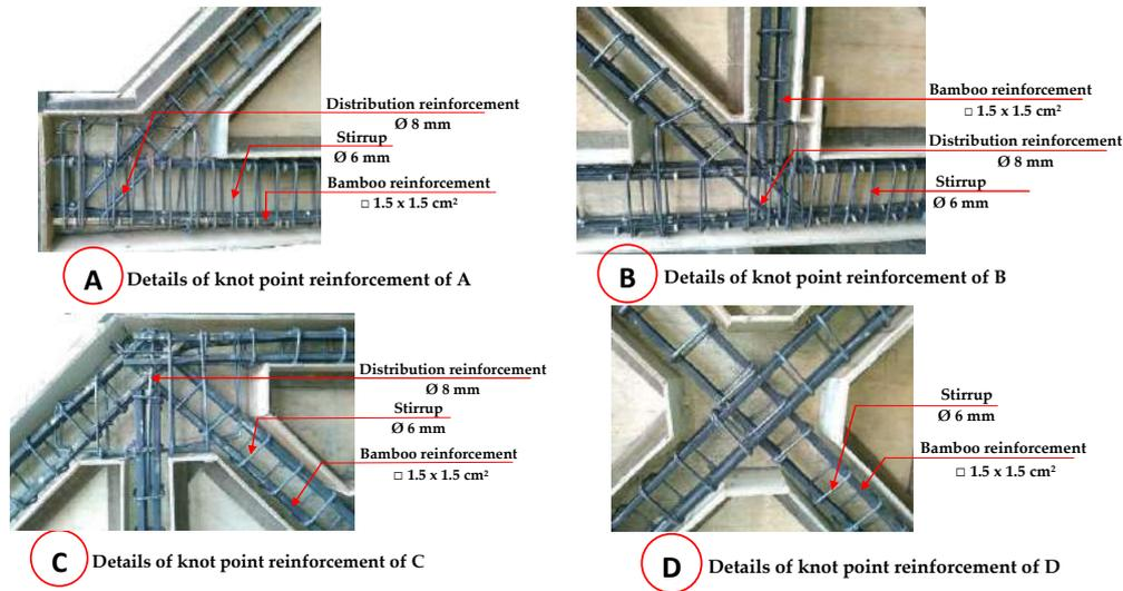
Figure 15. Details of the knot reinforcement for the bridge frames [38].
