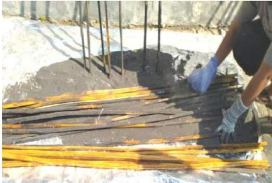
**Figure 7.** Sand sprinkling on bamboo reinforcement
