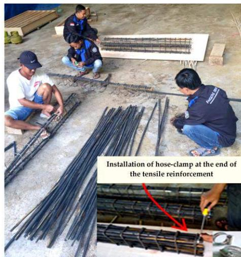
Figure 8. Stringing the bamboo reinforcement.
