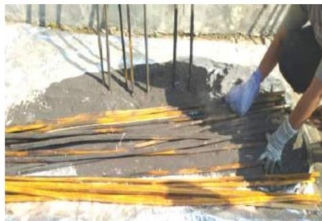
Figure 7. Sand sprinkling on bamboo reinforcement.
