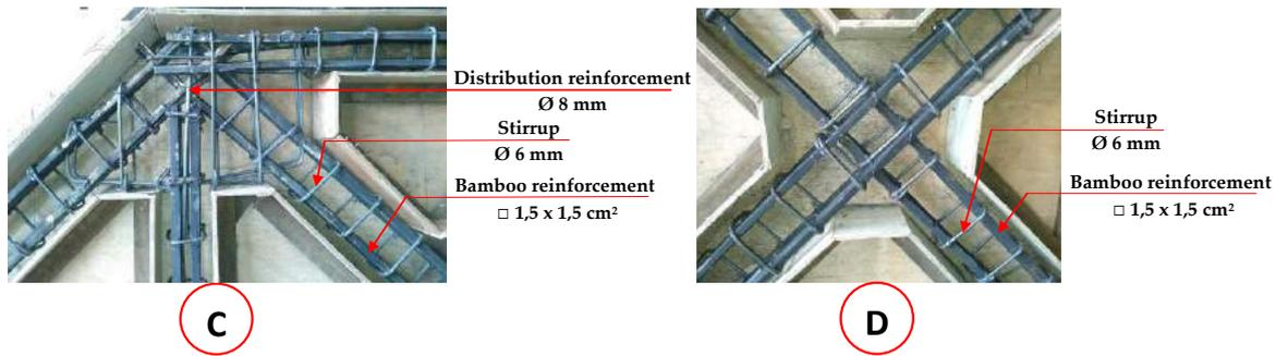
Figure 15. Details of knot reinforcement for bridge frames [23]
