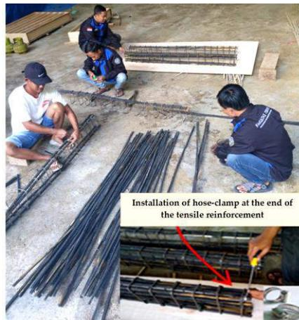
Figure 8. Stringing the bamboo reinforcement.
