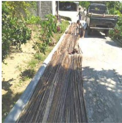
**Figure 4.** Drying bamboo in free air.
