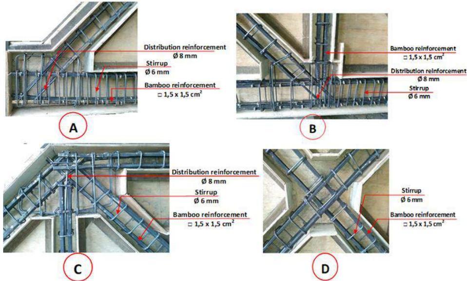
Figure 15. Details of knot reinforcement for bridge frames [23]
