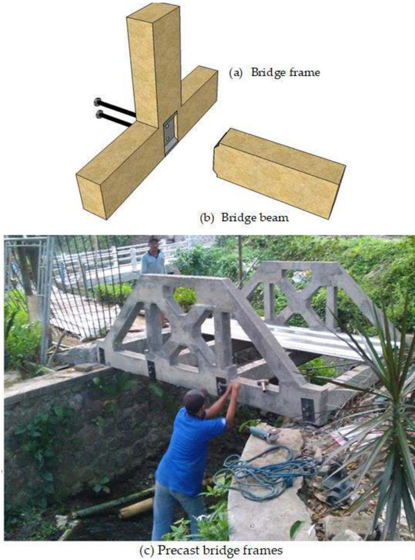
Figure 11. Models and applications of precast connections
