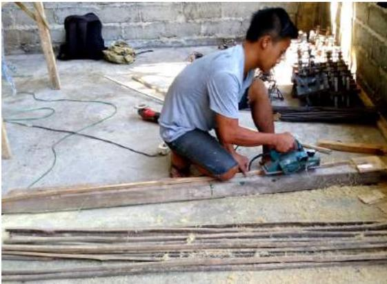
**Figure 5.** Tidy up the bamboo according to size
