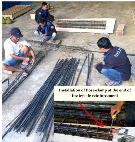
**Figure 8.** Stringing bamboo reinforcement
